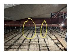
For the preferred new position we identified from the I-Beam to the ceiling, cable supports. These supports would have to be removed from the beam and transferred to another location or removed entirely if it is deemed safe. This is a request from North East Stage.
