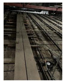
We also noticed the walking planks throughout to the preferred I-Beam making access to it much easier on both sides of the ceiling.
