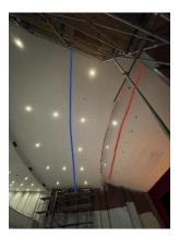
Red and blue lines are the locations of where the I-Beams are in the ceiling. The Red line is too close to the stage and not an optimal lighting position. The blue is where we need to go. From that beam it is 39' - 3" to the proscenium wall above the ceiling. From center stage to that location it is 58'. From the proscenium wall onstage 46'.
